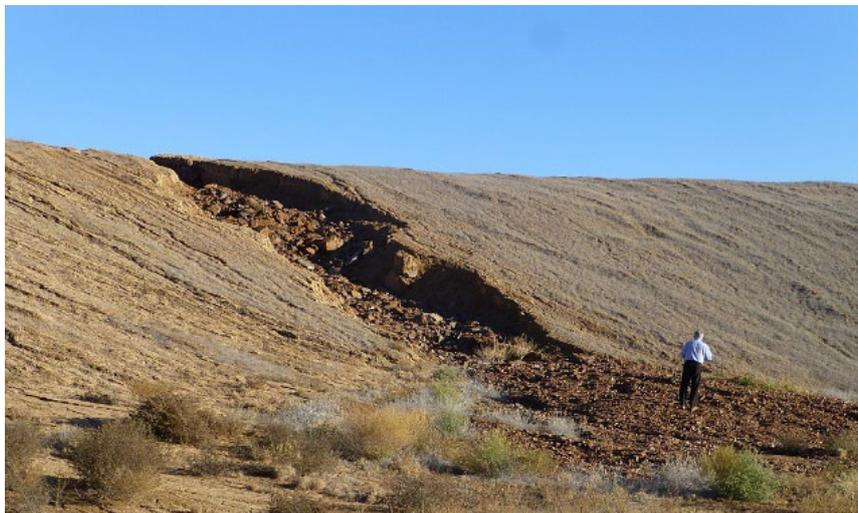
Image 1: Erosion gully on a uranium mine dump in southern Kazakhstan (BGR)
